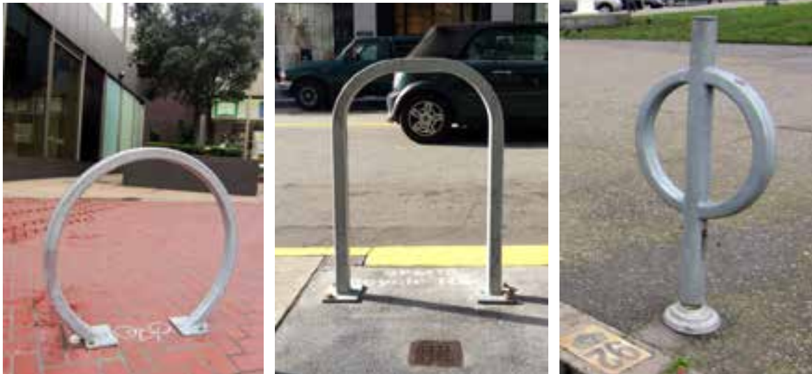
Figure 3 Short-Term Bicycle Parking in San Francisco (from left to right): Circular Rack (Standard Rack), Inverted U Rack (Previous Standard Rack), and Meter Post Ring
