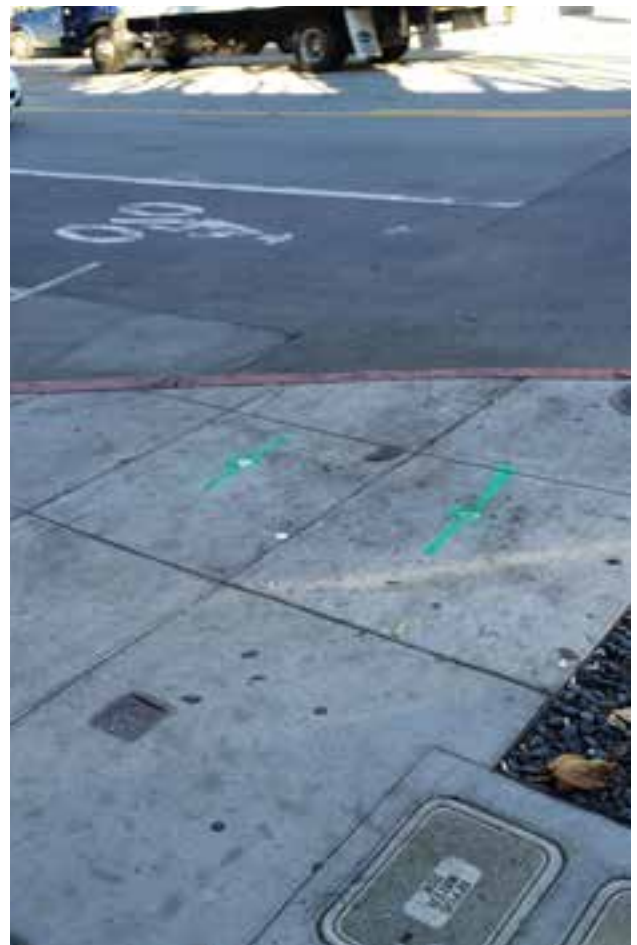
SFMTA staff paint the sidewalk with markings at approved locations.
